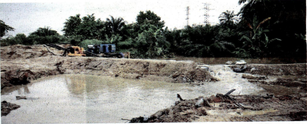
Work under way on the third bund at Kampung Sungai Buah, Dengkil, to prevent polluted water flowing into Sungai Langat, whose water is treated at the Sungai Semenyih treatment plant. — Picture by Mukhriz Hazim
